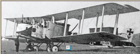
Another view of Ernst Brandenburg's Gotha built G.IV 624/16 at Nieumunster in May 1917. Details to note include the aircraft number 624 37 painted on the inner face of the wheels, anemometer mounted to the front left of the pilot and that the lower wing crosses appear to have white borders like 10 .
