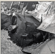
This view of crashed Gotha G.IV (LVG) 991/16 E shows the additional engine cooling louvers associated with LVG built G.IV engine nacelles. (Thomas Gentz)
